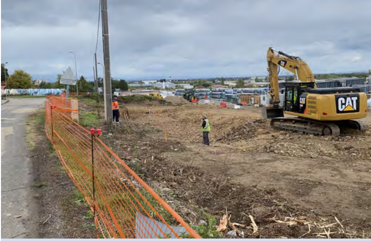
The start of the earthworks for the future unloading bays
